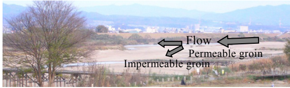
Photo 1 Groins along the Kizu River (positioning around 34°51'N and 135°44'E)
